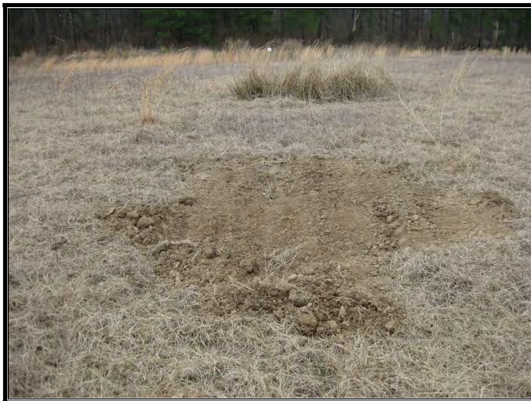
PHOTO 14: Repair of Holes in Landfill Cover DATE: February 1, 2019
