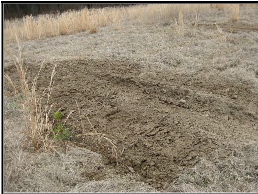
PHOTO 11: Repair of Holes in Cover DATE: February 1, 2019
